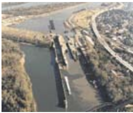
McAlpine Lock Project
