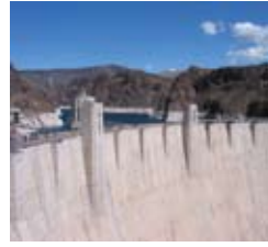
Hoover Dam Bypass Project
