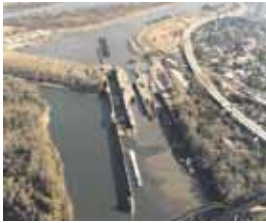
McAlpine Lock Project
