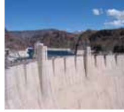
Hoover Dam Bypass Project
